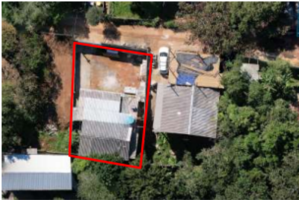
Figura 03 – Vistoria in loco .
